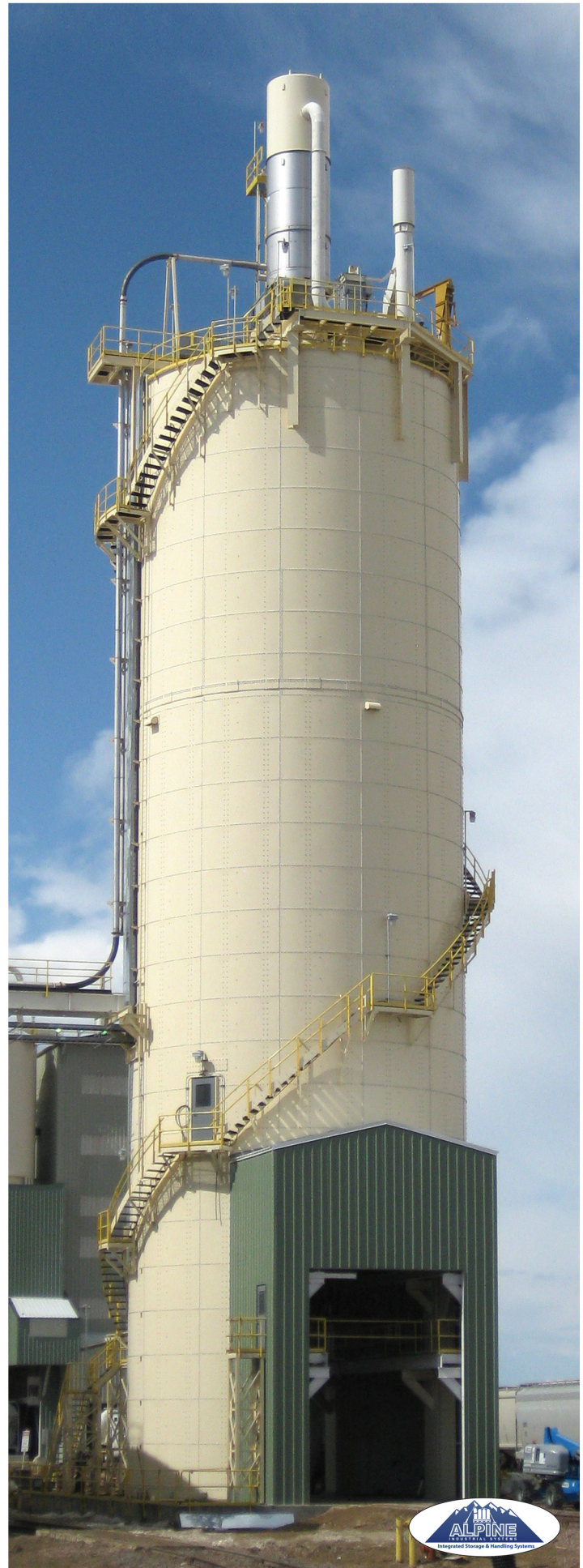
38' diameter x 130' tall fully skirted rail load out system
